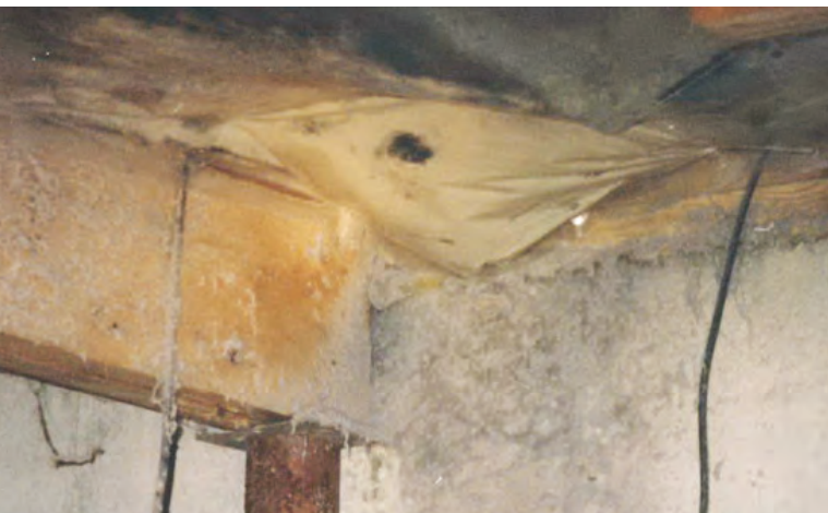
Lint from dryer vented into crawl space; moldy insulation was present. May Indoor Air Investigations LLC
