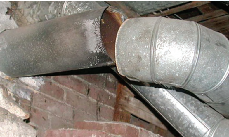
Fallen oil-furnace vent pipe in another house with unhealthy air May Indoor Air Investigations LLC
