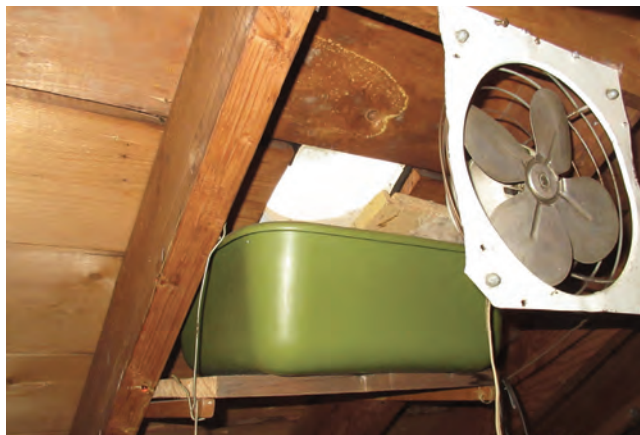
Photo 3. Attic Vent Pan and Fan
