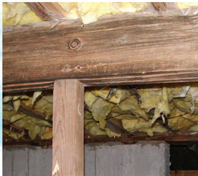
Beam decay due to moisture from dryer vented into crawl space. The top of the post penetrated the bottom of the decayed beam. May Indoor Air Investigations LLC
